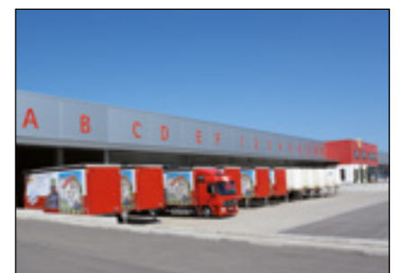
Teningen logistics centre
